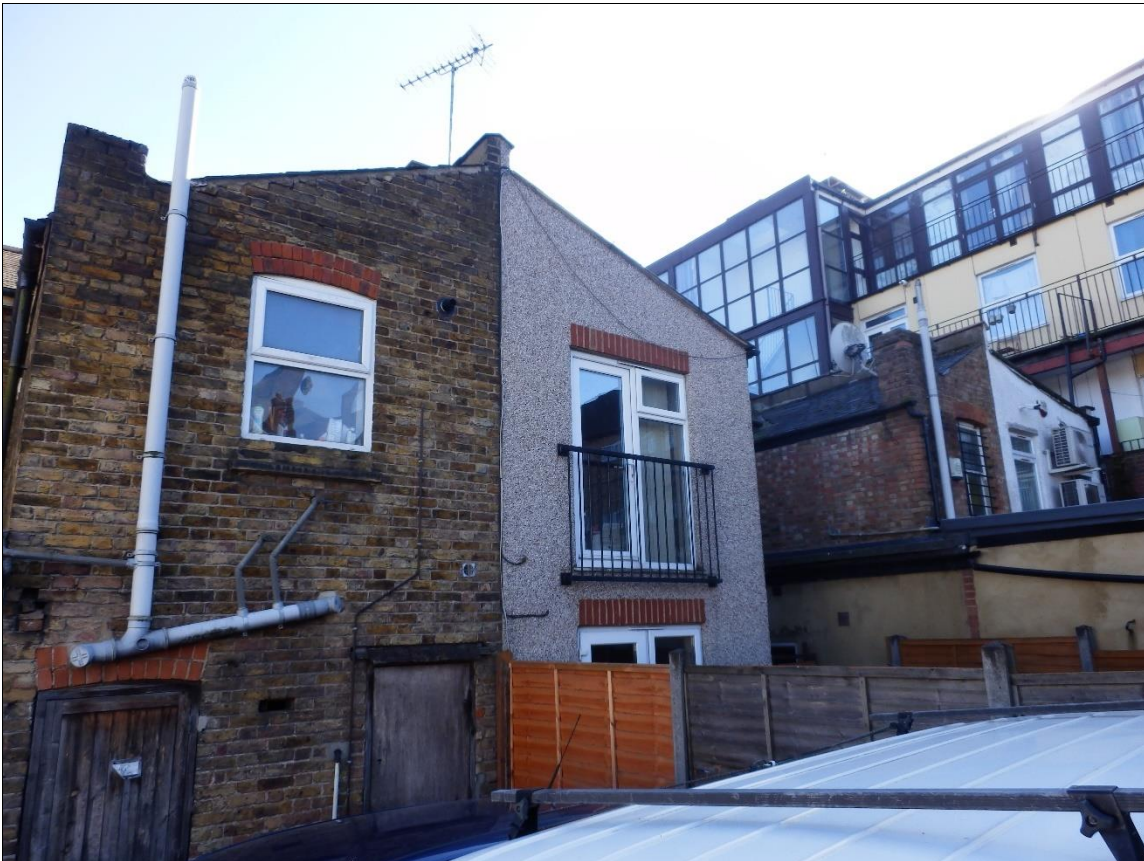
Rear of no. 14
