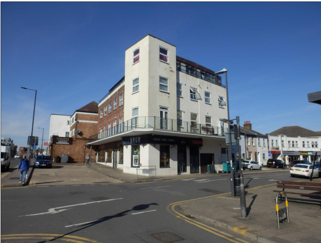
Looking towards site from Station Road
